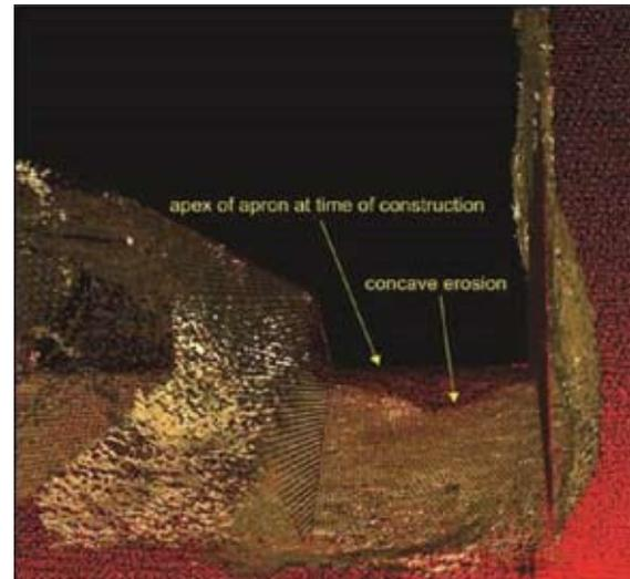
Fig. 5 : Hugh L. Keenleyside spillway - 3D sonar rendering of apron erosion between dissipators.
