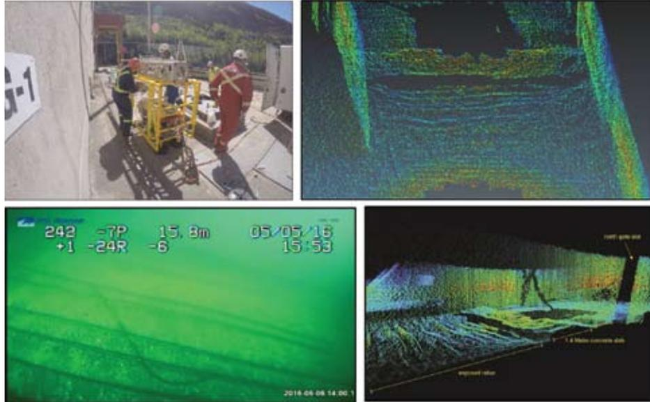
**Fig. 10** : Keenleyside Dam Spillway Surveys in BC, Canada. Clockwise from upper left: Site operations, 3D sonar rendering of exposed rebar on slab, same location from a different angle, and video
