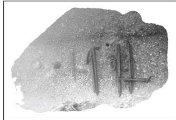
**Fig. 8 :** Photogram of dissipator pier erosion
