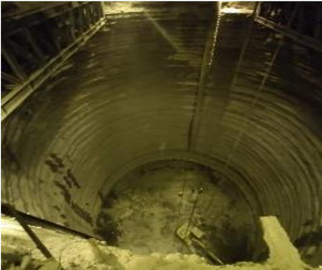
Fig. 13 : Excavated Portion of Both shaft with support
