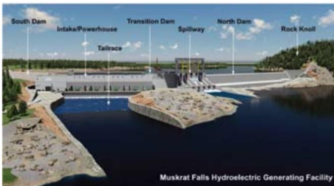
**Fig. 1 :** Muskrat Falls generation facility – Water retaining structures.
