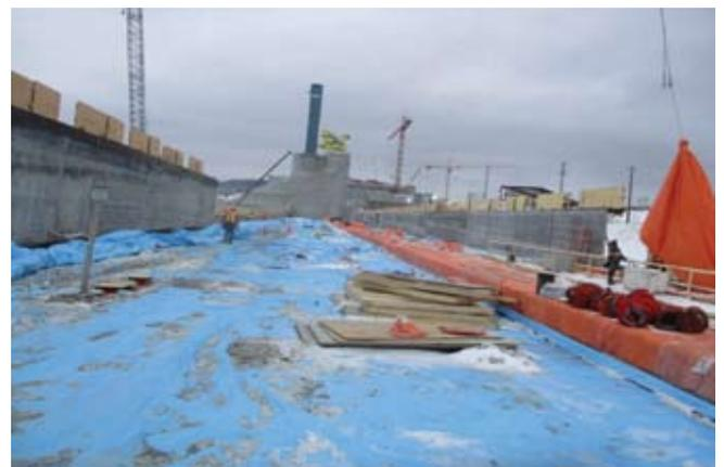
Fig. 17 : Insulated tarps on the North Dam at elevation 15.69 m
