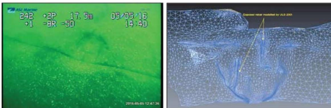
**Fig. 13 :** Video capture of eroded pocket in spillway (l) and the same location scanned with underwater laser (r).
